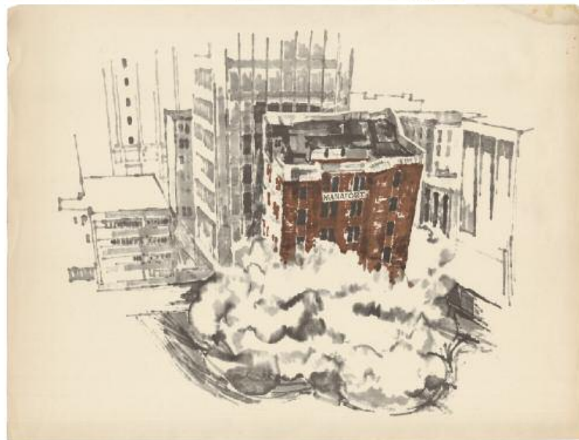
Demolition of the Judd Building, 75 Pearl Street. Photomechanical reproduction printed in black and brown ink, 1973. The headline in The Hartford Courant read "Blast Crumbles 9-Story Building in 9 Seconds," and the author of the article seemed to delight in the amazing new technology that made such speedy destruction possible. Welling's print appears to have been based on a photograph taken from the Hartford National Bank Building that appeared with the story.
